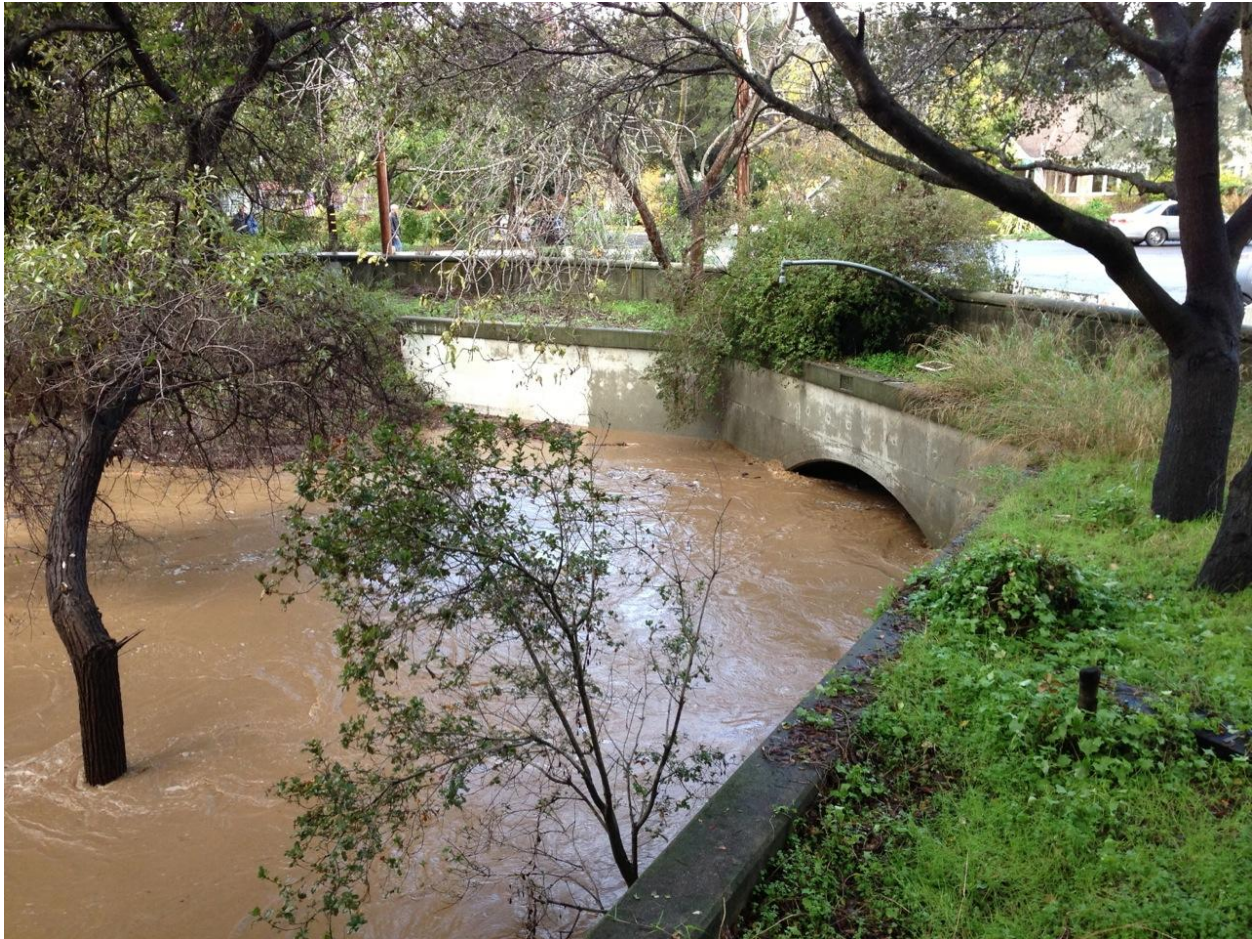
Figure 2 – Existing Culvert at Pope/Chaucer
